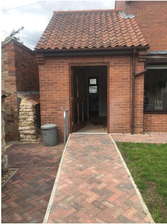
Ramp to side wheelchair entrance
